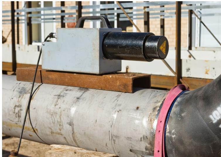
Figure 5: Non-destructive material testing - Inspection of weldings with a gamma ray source, Source: www.shutterstock.com .
